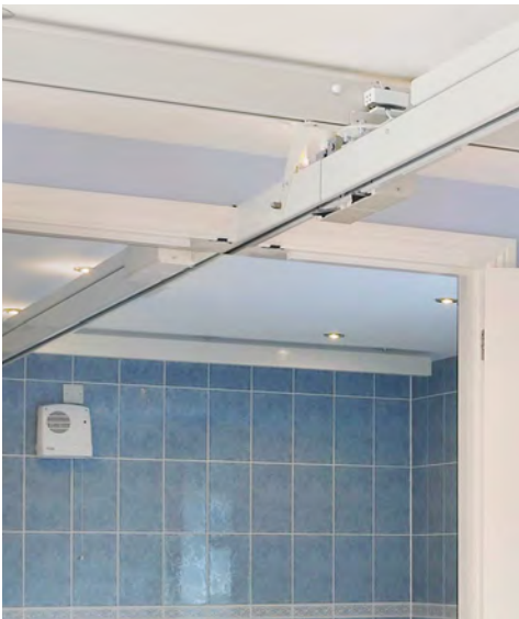
Two images showing a single track to transfer from the bed to the bathroom. Two different options for the track passing through a door header are shown.
