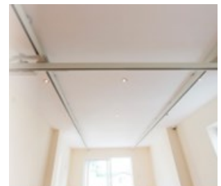
Large H-System covering the bath lounge and dining areas
